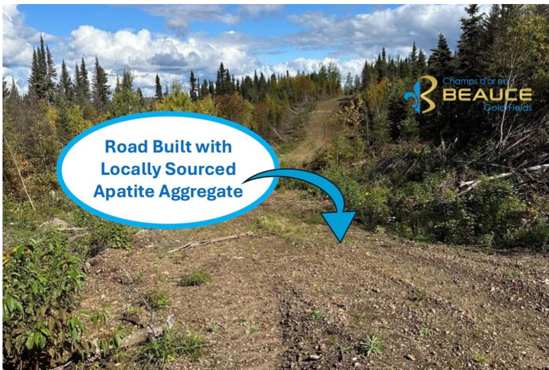
Apatite-bearing material was observed directly in road construction aggregate sourced locally
